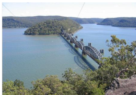
Hawkesbury River Railway Bridge alongside the piers of the original bridge. Source: Wikipedia .
