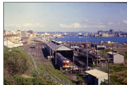
Newcastle East End Yard in 1985 with diesel multiple car sets prominent and an electric passenger car sitting isolated in the Yard. Source: David Patterson .
