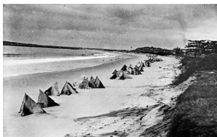
Primary beach defences in place backed by dune tank traps arising from a fear of Japanese attack on key Newcastle targets in WW2. Source: Flickr.
