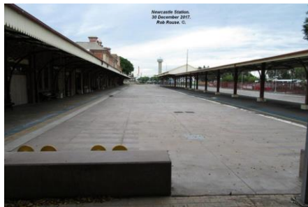
A lifted and levelled track surface at Newcastle Station in December 2017 with only symbolic buffers and a paved track outline remaining. Source: Rob Rouse.
