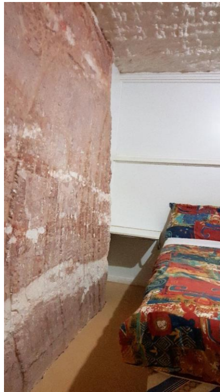
Riba’s Underground Accommodation – our room.
