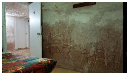
Riba’s Underground Accommodation – our room.
