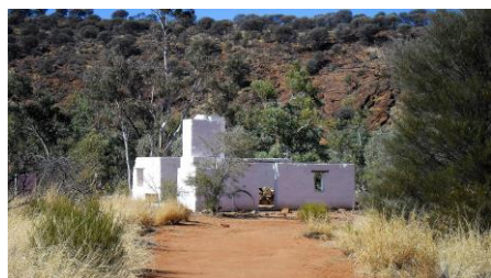
Old Owen Springs Station Homestead Ruin.
