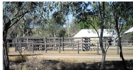
Outbuildings, Alice Springs Telegraph Station.
