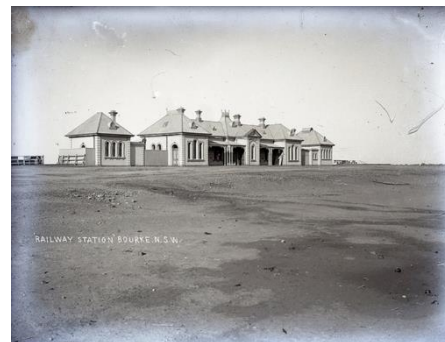
Bourke Railway Station built on a rise to protect from floods. Source: Flickr
