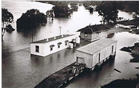
The Morgan Railway platform and wharf were covered with water, so a temporary platform was erected on the outskirts of Morgan, at Lanosa Siding.
