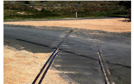
A triangle was eventually installed to turn locomotives being built too big to turn on the old turntable. The line at the top of this picture re-entered the main line to the L as described in top picture.
