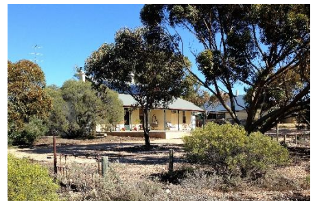
Former Railway Cottages facing NE.
