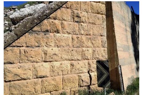
Railway bridge abutment – two tracks wide. Note the local stone used in its construction. Reinforced concrete was added to cope with the development of larger heavier freight cars and locomotives.
