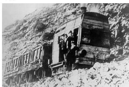
The 'Coffee Pot' locomotive hauling coal from the Glenrock Lagoon Colliery. Source: Flickr.
