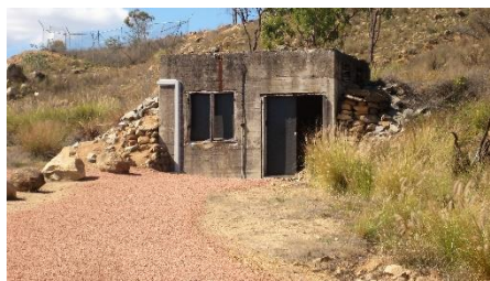
WWII bunkers scattered around Tower Hill.
