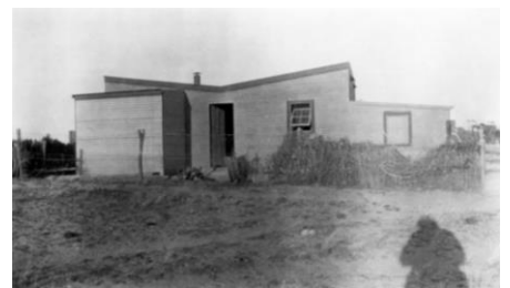
Puntabie Barracks, seen here in 1945, illustrates the corrugated iron construction of many early SAR barracks buildings. Rhonda Dorward.
