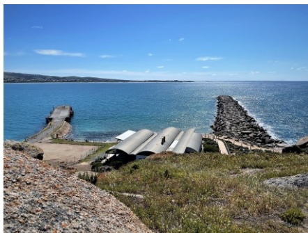
Access is available via the wooden stairway to the café area and pylon jetty. (Café currently not open).
