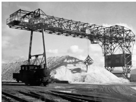
The yard shunter waits while the superphosphate crane takes another scoop at the Cockle Creek Works. Source: Newcastle Herald.
