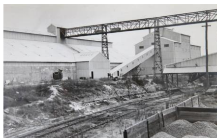
Polluted Pasminco sidings at Cockle Creek. Source: Newcastle Herald.
