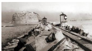
The causeway to Nobbys reinforced in later years by large rocks carried in by rail from the quarry at Waratah. Source: Newcastle Herald.
