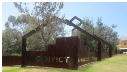
The Convict Lumber Yard site showing today's re-created symbolic memorial of the main building near Newcastle Railway Station and the former East End Railway Yard. From the 1860s, buildings including the Customs House, a Paymaster's building, a Sailor's Home and a residence for the Newcastle Stationmaster were built over the remnants of the Convict Stockade at the Lumberyard. Source: History Service NSW blog.
