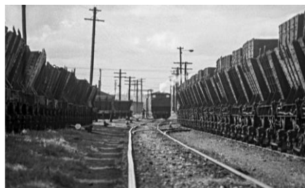
An SMR tank locomotive stopping for water amid lines of wooden coal hoppers. Source Mal Austin.
