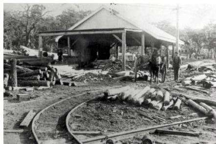
A sawmill at Catherine Hill Bay supplying the Wallarah Colliery with pit props in 1914 via an interesting arrangement with a tight narrow-gauge horse-drawn track crossing on top of a standard gauge line! Source: Newcastle Herald.
