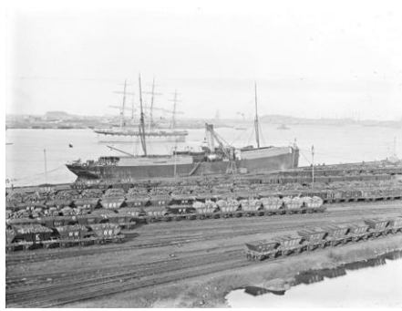
A steamer being loaded by a hydraulic crane at 'The Dyke' while a sailing ship stands off waiting its turn. Source: Newcastle Herald.
