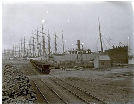
A full set of wagons waiting to be shunted to the hydraulic coal cranes at 'The Dyke' while a set of empties await picking up by a steam locomotive to run back to their colliery. Source: Newcastle Herald.
