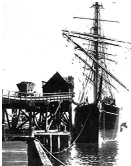
Loading coal at a Honeysuckle Wharf staithes on the South side of the Harbour in 1911. Source: Newcastle Herald .
