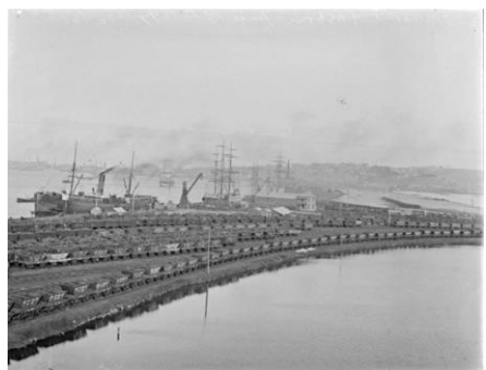
'The Dyke' chock-a-block with coal wagons waiting for their hoppers to be plucked by the hydraulic cranes. Source: PICCSR.
