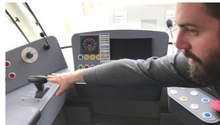
The driver’s main control stick including emergency stopping. The computer (near elbow) plays a significant part in the overall management of the unit, including lighting and temperature control.
