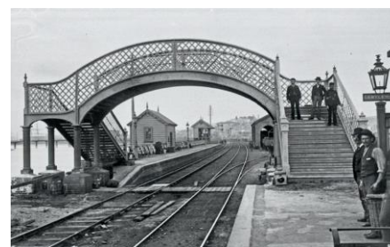
Honeysuckle Station with the bridge to Bullock Island, ‘The Dyke’ and Carrington in the background. The interesting opposing staggered platform arrangement was often used on the NSW Government Railways in the 19th century. Source: Newcastle Herald .
