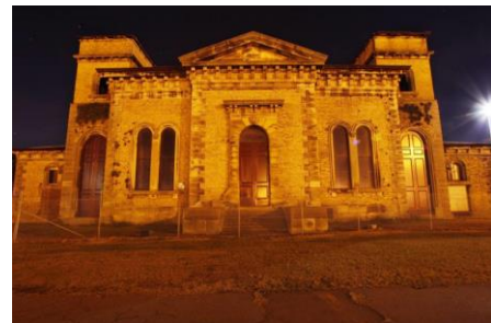
The impressive façade of the Carrington Hydraulic Pump House remains today like a temple from the past industrial age. Source: Newcastle Herald.
