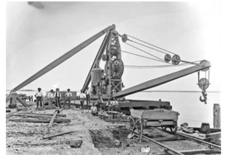
A work team with a 30-ton steam crane constructing rail and wharf facilities on the Dyke at Carrington in 1898. Source: Newcastle Herald.
