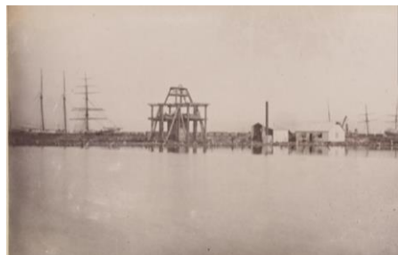
Sinking of a caisson shaft behind The Dyke to build the Hetton Colliery in 1877. Source: NSW Records.
