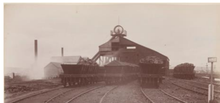
The Wickham Bullock Island Coal Mining Company rail yard. Source: NSW State Records
