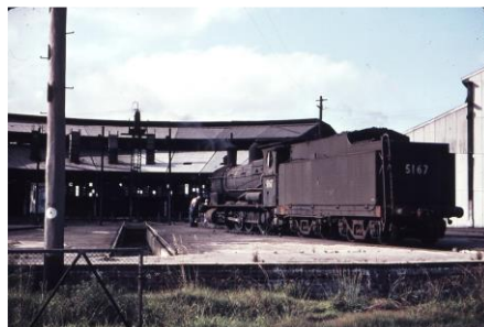
Port Waratah Locomotive Depot. Source: Weston Langford.
