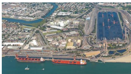
Port Waratah T1 Terminal. Source: Triplem .
