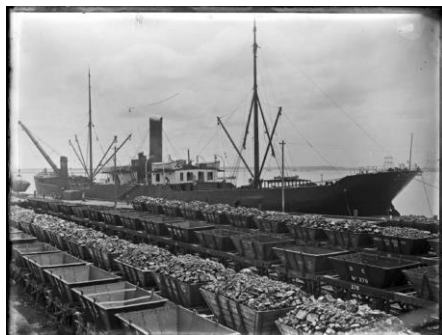
No 15 Hydraulic crane run from a steam driven hydraulic pump house loading coal at 'The Dyke' in 1904 by lifting wooden coal hoppers from their fixed four-wheel bogies. Source: Newcastle Herald.
