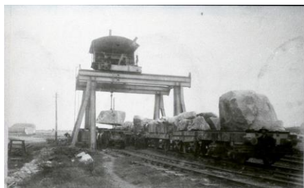
Construction of the Northern Breakwater at Stockton. Source: Newcastle Herald.
