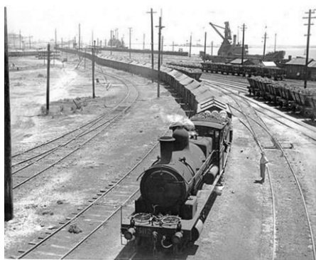
Grain train passing through The Dyke coal yard on Carrington in 1947. Source: Newcastle Herald.
