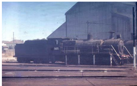
Loco 5475 waiting at Port Waratah Loco Depot and Turntable. Source: NSWrailrambler.
