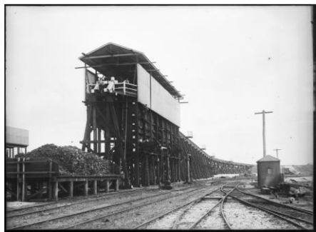
The finished Port Waratah Coal Stage. Source: Flickr.
