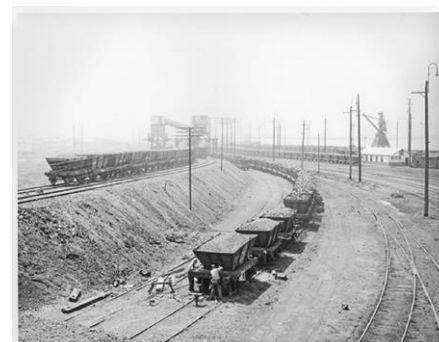
The Dyke Railway Yard at Carrington. Source: Newcastle Herald.
