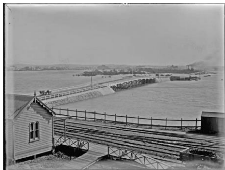
Looking across from Honeysuckle Station on the Newcastle Station Branch across to Bullock Island Bridge and its collieries in 1900. Source: Newcastle Herald.
