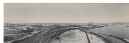
The Dyke on the seaward side and The Basin to the right with the Hydraulic Pump House in the middle of the network of railway lines in 1904. Source: NSW Library
