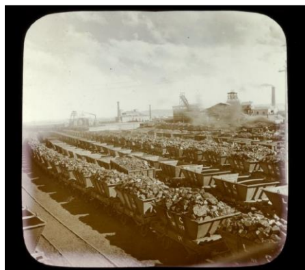
Bullock Island (Carrington) with coal wagons and the two collieries in the background and the Hydraulic Pump House in the middle to drive the loading cranes on The Dyke. Source: State Library of Victoria.
