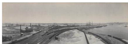
The Dyke on the seaward side and The Basin to the right with the Hydraulic Pump House in the middle of the network of railway lines in 1904. Source: NSW Library
