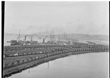
Crowded coal loading at No. 11 hydraulic crane in 1897. Source: Newcastle Herald.
