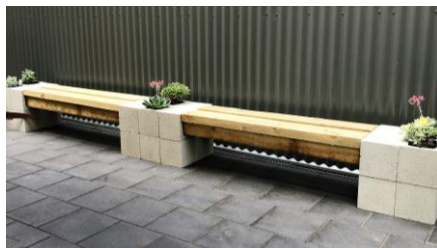
Four vertical, recycled Permapine beams inserted into the Besser/Cinder blocks and horizontal planks screwed to the beams. No glue used. Each seats 2 to 3 people. Quite sturdy.
