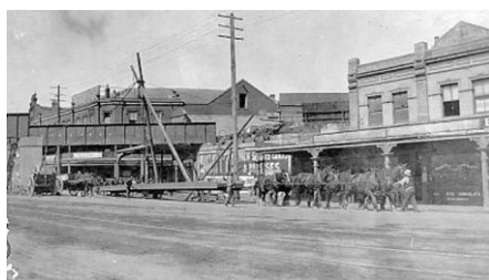
Dismantling of the 1865 iron bridge with horsepower in 1921. In the 19th century the bridge marked the boundary of the city and A.A. Company 2,000 acres of coal land it received in a Government grant. Source: Newcastle Library.
