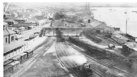
A busy Newcastle Station Yard in 1879. Source: Newcastle Herald.
