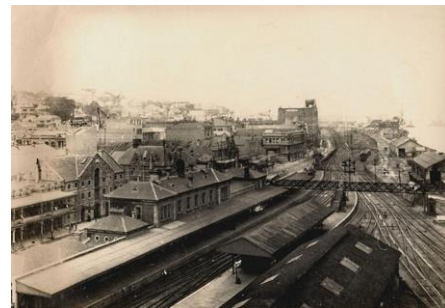
Newcastle Station squeezed between the city and the Harbour and part of a 160-year argument. Source: Flickr.
