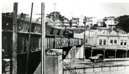
Coal wagons being hauled across the AA Co's bridge in its last years. Source: Newcastle Herald.
