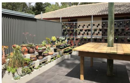
Closer view of the table using recycled Permapine for the main frame. Permapine posts were used in the end instead of Besser/Cinder blocks.
