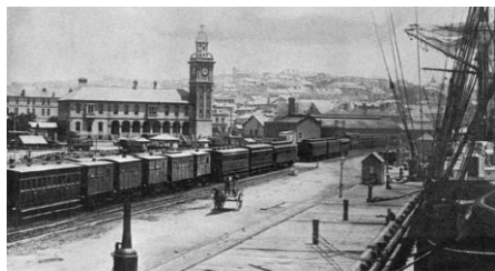
Passenger cars waiting for duty in the Newcastle Station Yard adjacent to Queen's Wharf. The photo was taken ambitiously from a sailing ship's rigging with the chimney of a steam crane below. Source: Newcastle Herald.
