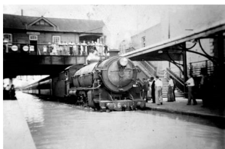
A 36 class-hauled train waits to depart Maitland Station during the 1955 Flood. Source: Cessnock Advertiser .
