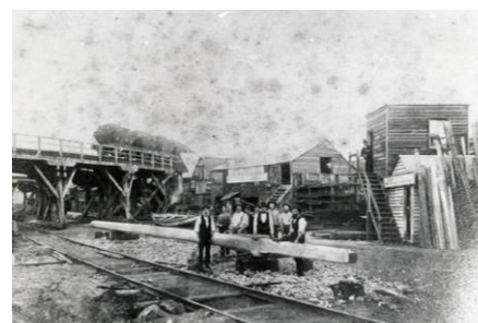
Workers preparing timbers for extending the AA Company’s coal loading staithes running to the dockside. Source: Newcastle Herald .
