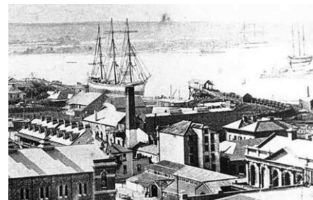
Burwood Colliery coal loader with a series of wagons on the staithes with an open-sided shed running out over the water. Source: NIHA.
