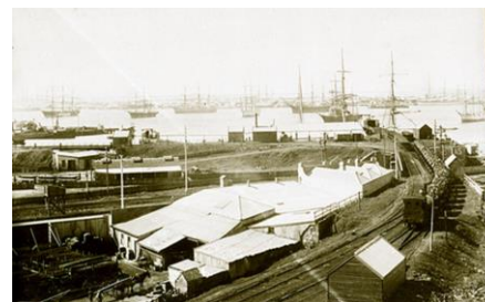
AA Company wooden hopper wagons full of coal being pushed along the loading staithes to a waiting queue of ships. Source: Flickr .
