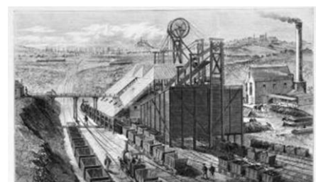
NAA Co mine in 1875, with the ships' masts in the distance. Source: State Library of Victoria.
