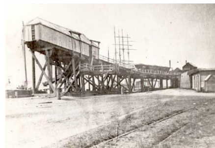
The AA Company coal staithes at Kings Wharf near Honeysuckle Station (later Civic Station precinct). Source: Newcastle Herald .
