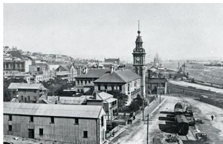
The ball on the Customs House spire was raised approaching 1pm each day to be dropped right on the hour so officers aboard ships in the Harbour could set their chronometers. Source: Bing Images.
