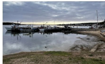
Coffin Bay - Main Jetty.
