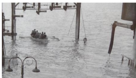
A flood boat being rowed under the Maitland Railway Station signal gantry in 1955. Source: ARHS .
