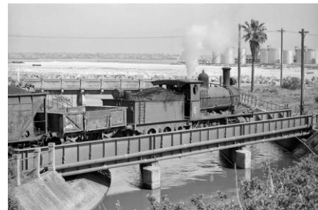
Boiler ash train at Bunnerong Power Station in 1973 heading towards the sandy dune country. Source: Flickr.
