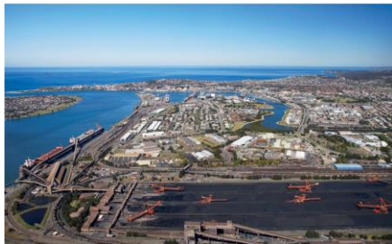
Port Waratah Coal Loaders feeding coal from rail-fed dumps into ships. Source: Sierra Club.
