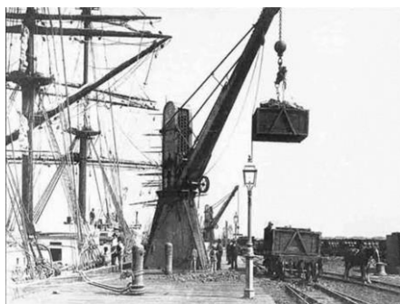
A coal hopper being lifted from the wagon frame by a hydraulic crane to swing over the ship for the floor release to be opened and coal tumble into the hold. There was an energy mix of steam power for the rail locomotives and Hydraulic Pump House, horsepower for shunting wagons, and gas power for wharf illumination. Source: NIHA .
