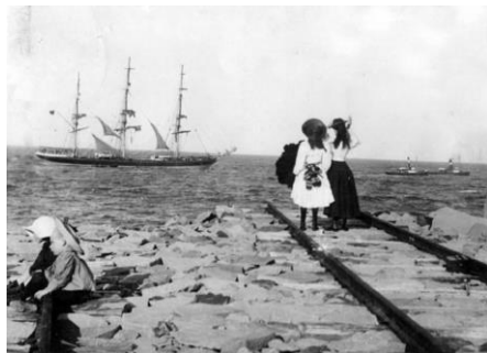
Girls on Macquarie Northern Entrance Breakwater being extended c1900 waving to a passing sailing ship being led by dual steam tugs. The lack of buffers preventing a drop off into the ocean was unnerving! Source: Newcastle Herald.
