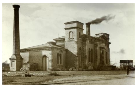
The Hydraulic Pump House with its twin chimneys and water tower (the chimneys and tower are now demolished). Source: Discover the Port .
