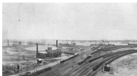
An indication of the scale of the port investment in Newcastle at Hamilton Junction’s spurs to ‘The Dyke’ on the left, Newcastle Station Precinct and Nobbys on the right, and the Great Northern Line to Broadmeadow at the bottom. In the centre is Carrington Hydraulic Pump House in 1904. Source: ABC .
