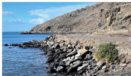
Bluff Jetty Road.
