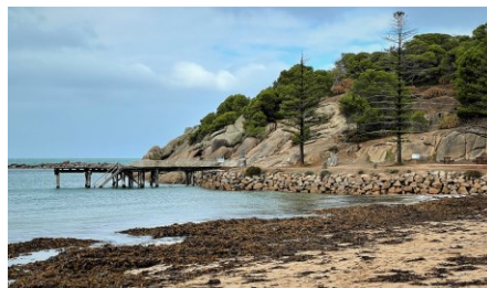
Port Elliot Jetty.
