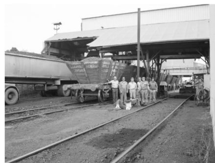
The last wooden hoppers dumping at the Hexham Coal Preparation Plant in 1987. Source: University of Newcastle.
