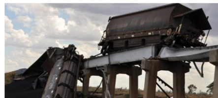
Sometimes not everything goes according to plan. In 2012, a fully laden coal train derailed just South of Boggabri and five wagons plunged off a bridge. Fortunately, nobody was injured. Source: Australian Journal of Mining.
