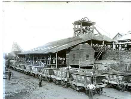
The 19th century Newcastle Mining Company grading and load out facility for wooden rail hoppers in the short coal chain to the Port of Newcastle. Source: Newcastle Herald.
