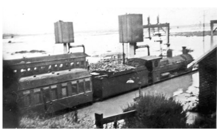
Floods at Maitland Station in 1955. Source: Flickr.
