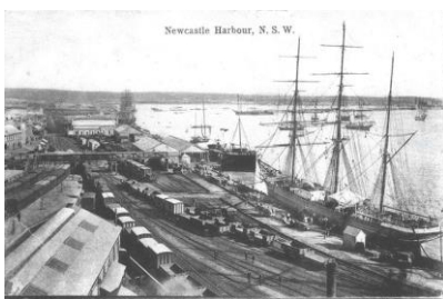
A busy Newcastle Railway Precinct c1870s with the passenger platforms on the mid-left and the East End Marshalling Yard in the centre and 'The Dyke' being constructed in the mid-right background. Source: Newcastle Herald .
