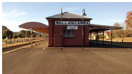
Wallangarra Station with the narrow-gauge track on the left and the standard-gauge on the right with accompanying awnings. Source: Garry Reynolds.
