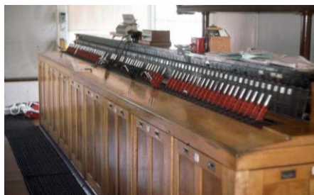
Newcastle Box signal frame, 1985. Source: Graeme Skeet.
