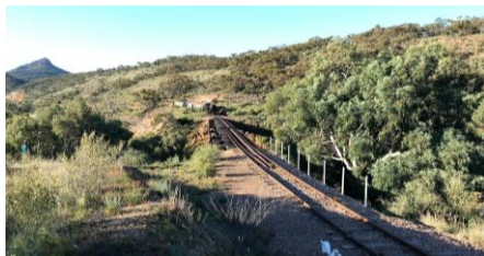
Woolshed Flat Bridge looking toward The Devils Peak .
