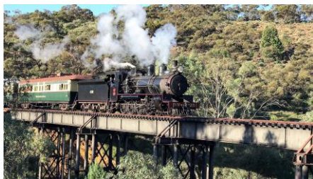
Woolshed Flat Bridge.
