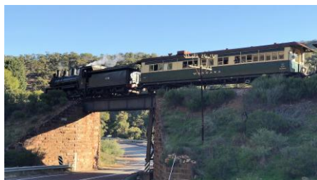
S-Bend Bridge looking south west.
