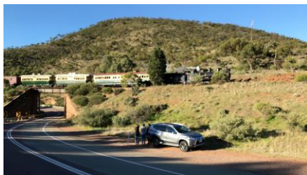
S-Bend Bridge looking north east.
