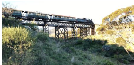
Lattice Girder Bridge.
