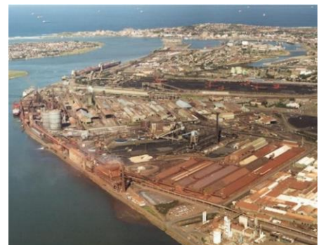
The sprawling BHP Steelworks dominated the landscape and the City of Newcastle. Source: NIHA.
