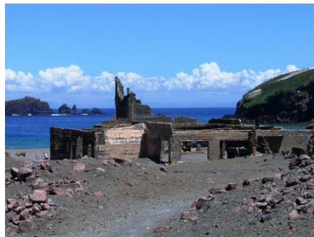
Another view of a 1920s sulphur processing plant.
