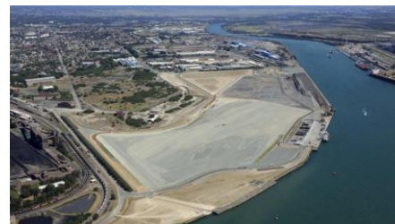
The BHP Steelworks site cleared. Source: Newcastle Herald.
