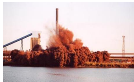
Demolition at BHP Newcastle. Source: NIHA.
