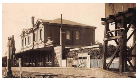
Moss Vale Railway Station where the line from Unanderra met the Main South Line. Source: Flickr .
