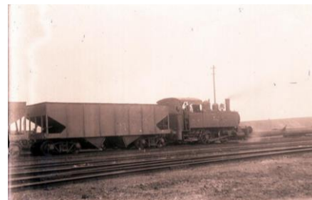
The 'Little Engine that Could' at the Newcastle Steelworks. Source: Flickr .
