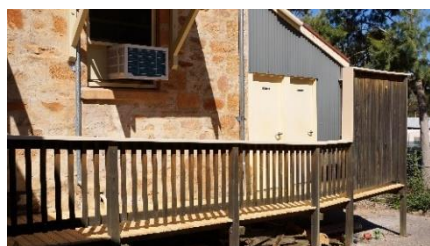
The floor of the toilet walkway has been renovated as well. ***
