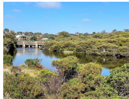
Railway bridge over Hindmarsh River viewed from the beach.
