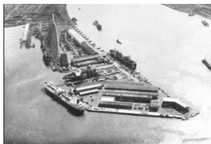
Plate 17: Aerial view of State Dockyard September 1945 The State Dockyard Newcastle NSW, 1945
