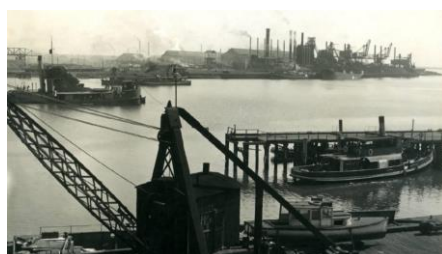
Steam dredges excavating the Hunter River channels between the Steelworks and the Dockyard in the foreground. Source: Newcastle Herald.
