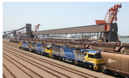
Port Waratah Coal Loading Terminal. Source: Rusted2theRails.
