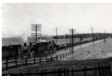
The vulnerability of the coal, rail and shipping industries in the Hunter to severe weather has always been a challenge. A goods train tiptoes through the waters in the 1995 Maitland Floods. Source: Hiveminer .
