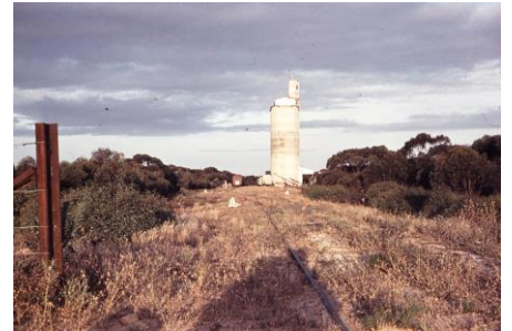
105324 Peebinga Up end Looking East.
