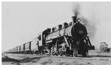
Example of an ore train used on Eyre Peninsula, SA.
