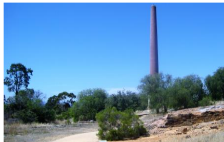
Beehive Company Mine Chimney, Maldon, Vic.
