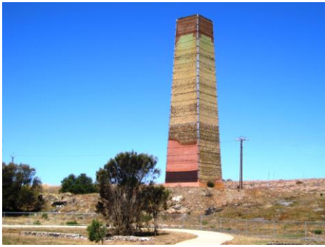
Smelter Chimney, Wallaroo, SA.
