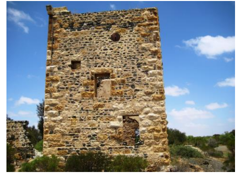
Pump House, Wallaroo Mines, Kadina, SA.
