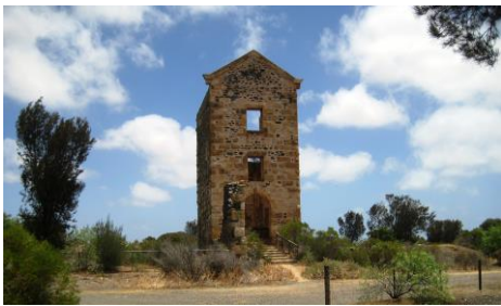
Pump House, Wallaroo Mines, Kadina, SA.
