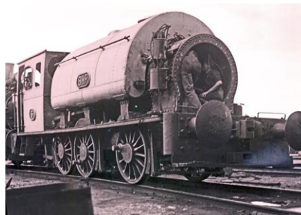
Undertaking running repairs to BHP Saddle Tank Locomotive No.6 at Newcastle Steelworks. Source: University of Newcastle.
