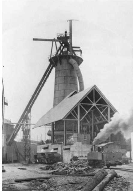
BHP Newcastle's first blast furnace with the slag pots on the side of the furnace and steam loco waiting while they are being loaded with slag. Source: NIHA.
