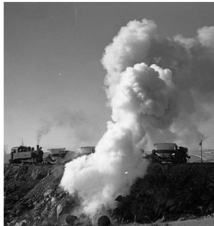
Tipping slag at Mayfield. Source: University of Newcastle.
