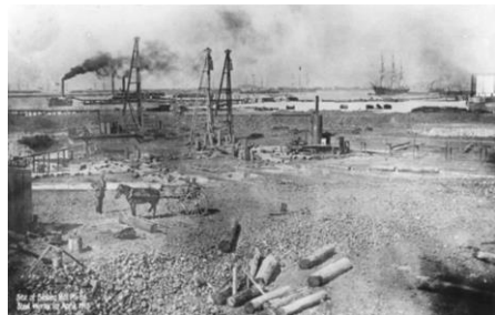
Constructing the BHP Steelworks in the era of the horse, steam and sail. Source: NIHA.
