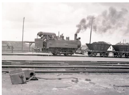
BHP Newcastle Tank Locomotive No.17 hauling coal wagons from the Borehole Colliery. Source: Flickr.
