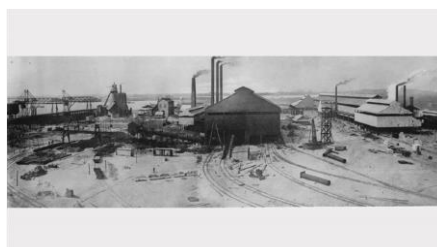
Early days of the BHP Steelworks built on mud and sand dredged from the Newcastle Harbour with the plant linked by a network of railway lines. Source: Newcastle Herald.
