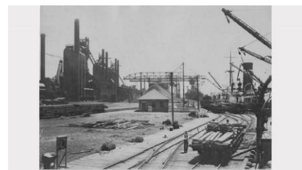
The ship-loading wharf at BHP Newcastle with accompanying rail lines. Source: Newcastle Herald.
