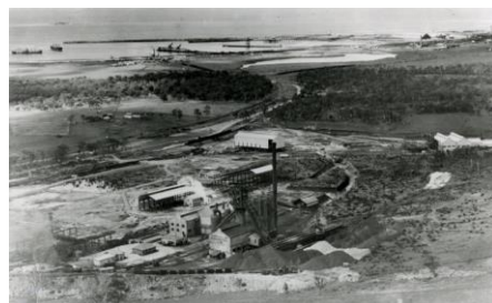
The AIS Port Kembla Steelworks being constructed. Source: Illawarra Mercury.
