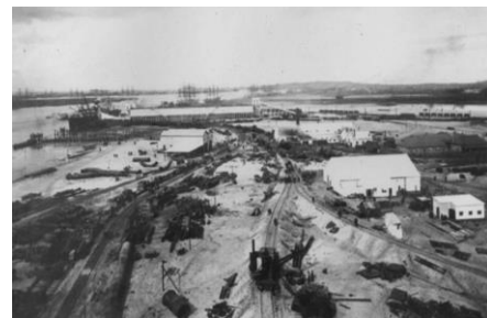
Construction of the Steelworks well underway with a network of railways. Source: Heritage Hunter.
