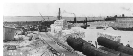
A construction railway threads its way through the Newcastle Blast Furnace at the BHP Steelworks site. While the latest technology was being installed by BHP, it was still an era where coal carrying sailing ships were moored at the Stockton Ballast Grounds in the distance. Source: Newcastle Herald.
