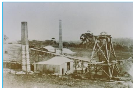
Bird in Hand Mine 1884. View looking west towards Winding House with tramway to Twenty Head Stamp Battery.
