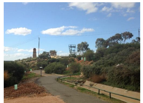
Heading along the 90-foot channel toward the cliff-top lookout.
