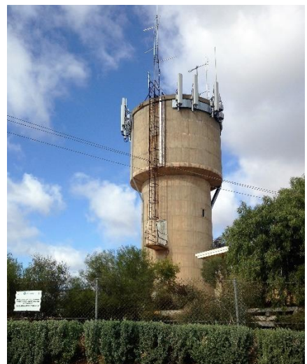
Waikerie water tank.
