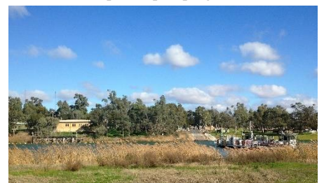
Today's - Waikerie Pumping Station and Ferry. ***
