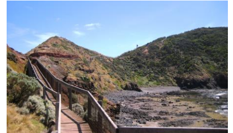
Boardwalk, Cape Schanck Lighthouse, Vic.
