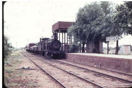
19 class locomotive hauling a mixed into Byrock on the way to Bourke. Source: Bing Images .
