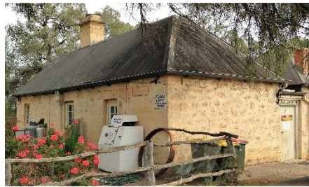
Note the 1956 flood level marker.
