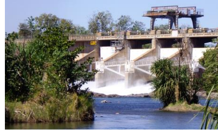
Weir for the Ord River, Kununurra, W.A.
