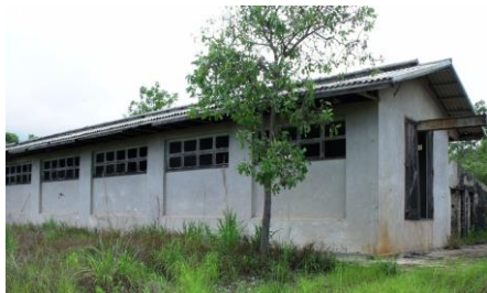
Top secret laboratory at Snake Creek (this building was even air-conditioned, and had gantries for moving shells).
