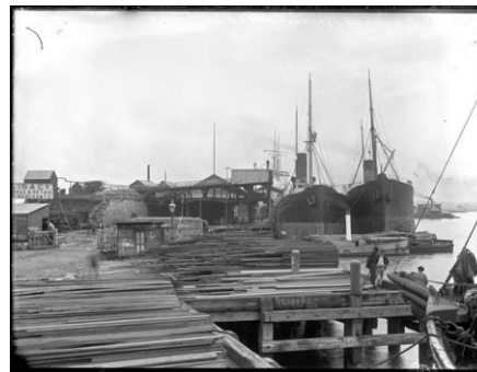
The AA Co wharf with a railway-fed coal loading staithe for ships in 1897. Source: Uni of Newcastle .
