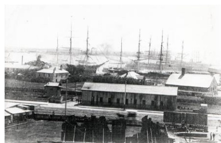
The original Newcastle steam tram sheds in the foreground with the railway running along the wharf feeding the ships with coal at Kings Wharf surrounded by an assortment of AA Co buildings. Source: Newcastle Herald .
