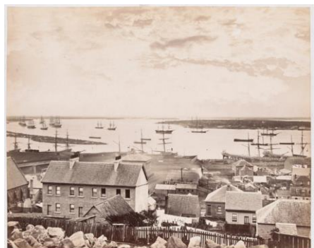
Newcastle Harbour in 1875 with "The Dyke" (left centre) at Carrington being built from offloaded sailing ship rock ballast from around the world and Stockton to the right with ballast grounds as well. The Great Northern Railway runs along the foreshore to Newcastle Railway Station and marshalling yard – all closed today. Source: State Library of Victoria.
