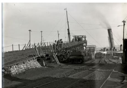
Stockton Colliery railway coal loading staithe. Source: Flickr.
