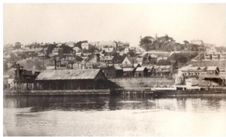
The Newcastle Boat Harbour and a coal staithe for loading ships from rail coal wagons. Source: Newcastle Historical Society.
