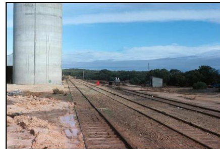
Picture of Peebinga railway siding taken before the line closed in 1990. Source: Internet
