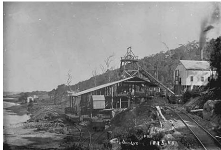
Burwood Colliery at Glenrock Lagoon in 1885. Source: NIHA.
