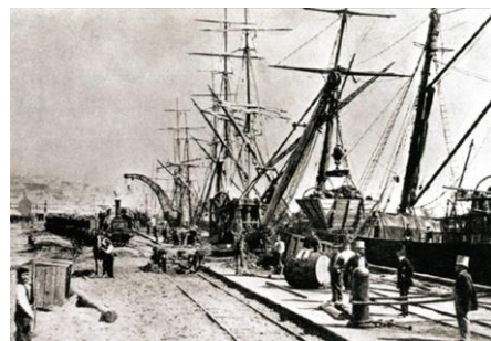
Queens Wharf near the Pilot Station in the 1860s loading coal with steam cranes. Source: The Herald.
