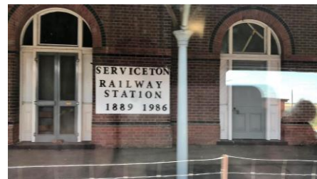
Serviceton Railway Station – long-time locked-up.
