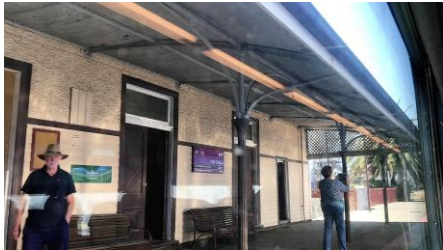
Nhill Railway Station...still in service.
