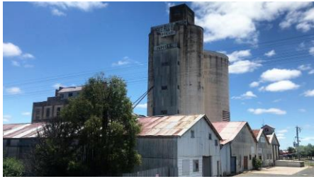
A very large, old flour mill and grain silo...Noske Flour, Nhill, Victoria. The Noske Silo at Nhill is the largest single bin silo in Australia.
